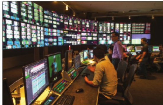
In the new Mediacorp Campus, the Media Operations Centre leverages IP to interconnect different broadcast systems for the transmission of audio and video content. SDI, however, is still deployed in many of Mediacorp's workflows.
